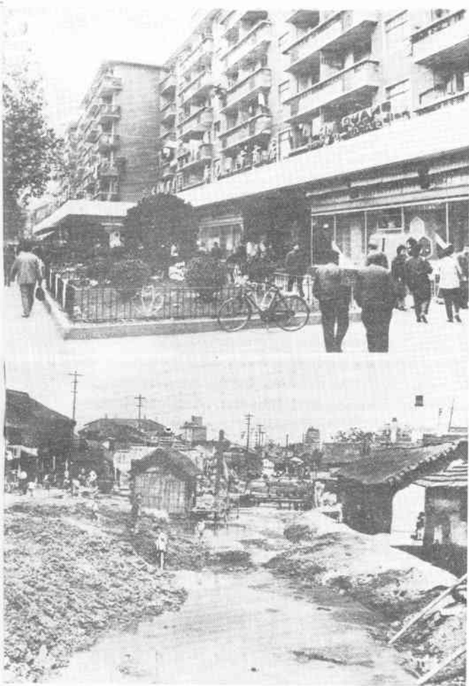
The modern Xianghua Street (above) was built on what used to be a stinking, dirty ditch (below) in Shanghai.
