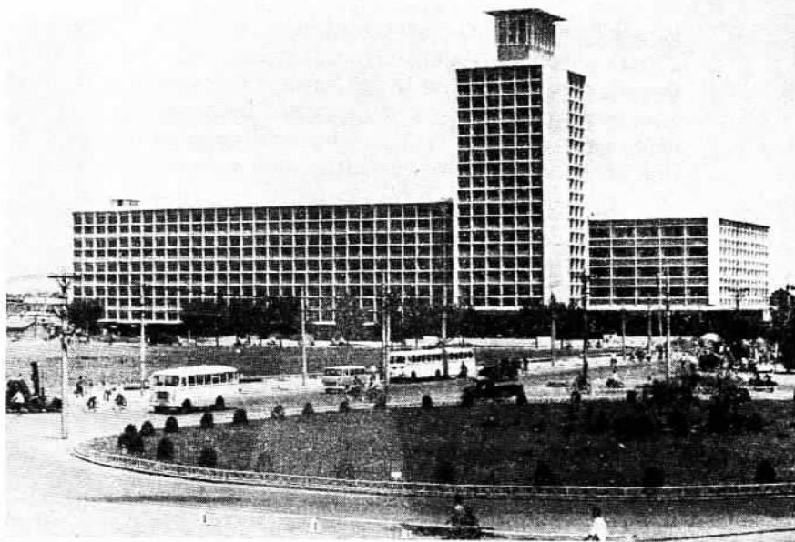
The telecommunications building in Shenyang.
