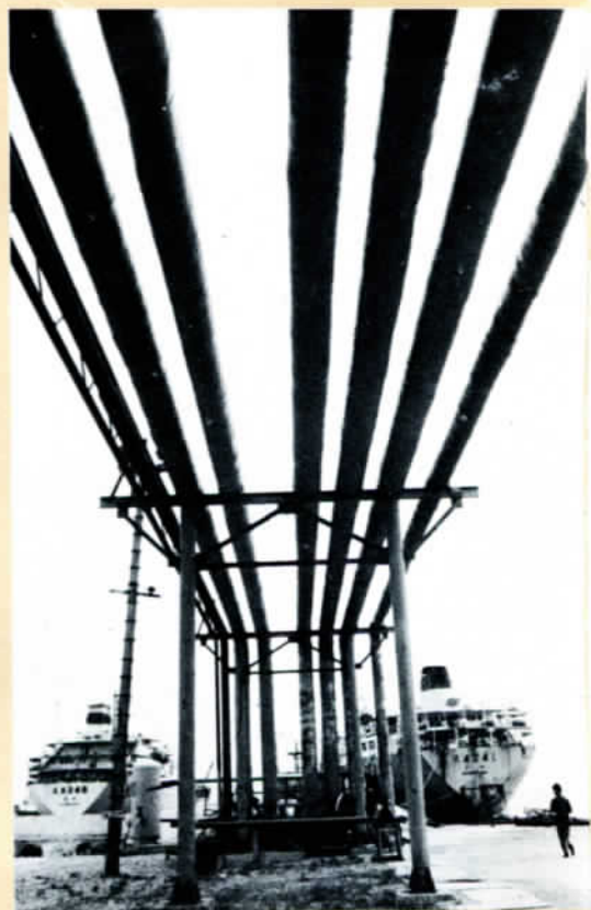
China's first mechanized oil wharf is being rebuilt.
