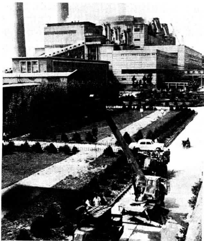
The Shentou Power Plant — the biggest thermal power plant in Shanxi.
