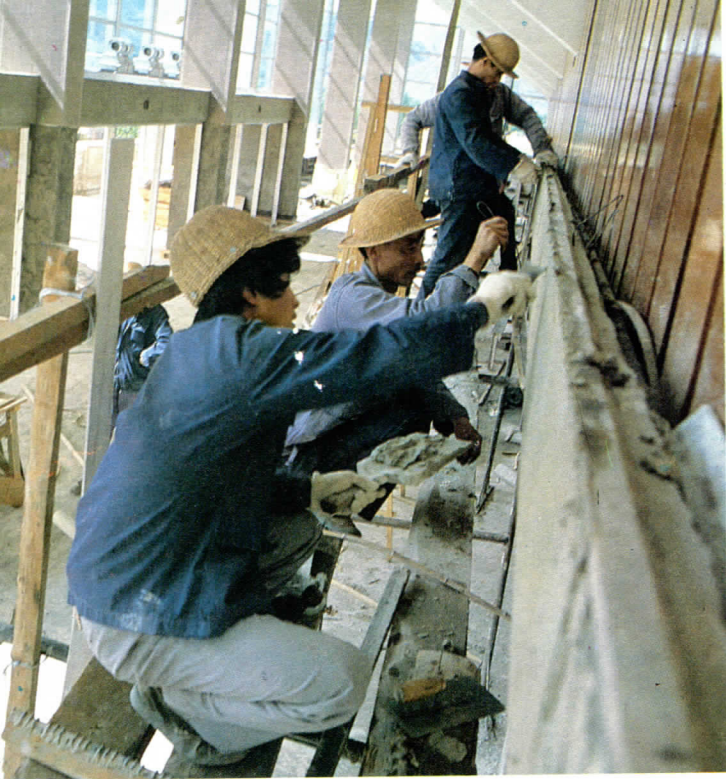
Construction progresses on the Qinghai-Tibet Plateau.
