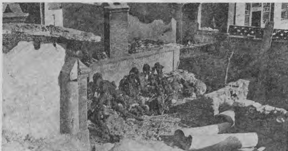
Panchiayu, a Hopei village, was completely wiped out with its 1035 inhabitants.
