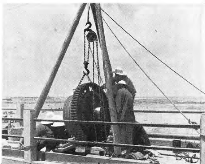
Installing electrical equipment to control the sluice gates of the dam
