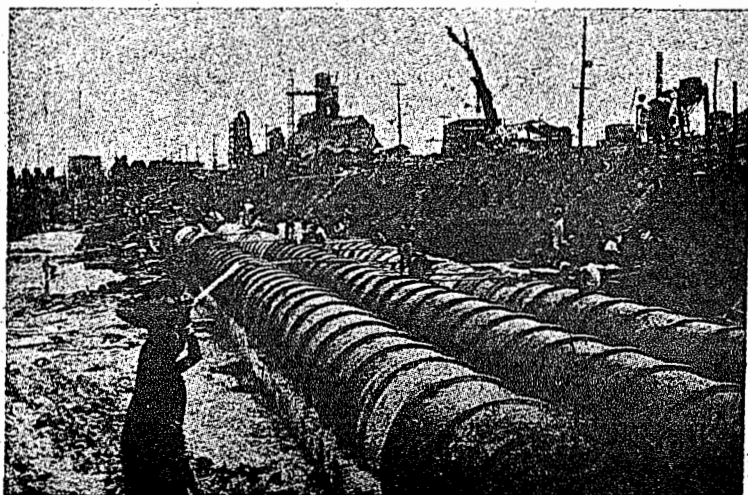
AT THE CONSTRUCTION SITE IN BHILAI
