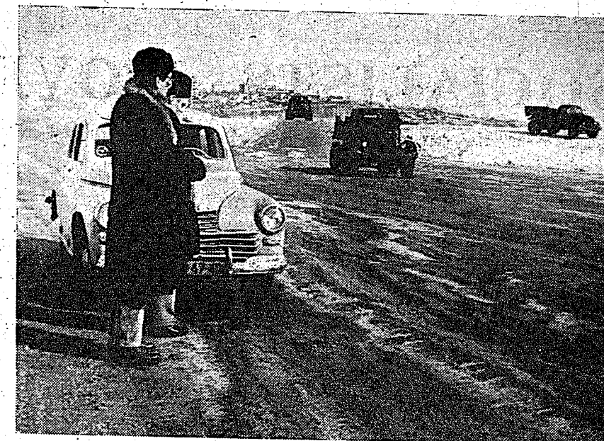
At Khabarovsk. It is on the five-foot-thick ice over the great river of the Far East, Amur, that the trucks and cars—and even excavators—are rolling across.
