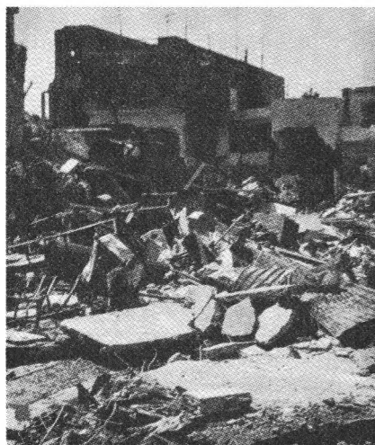
Destruction in Sabra
