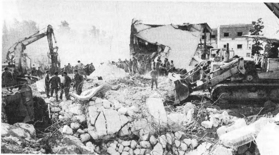
Ruins of Israeli military base in Tyre destroyed by the resistance.
