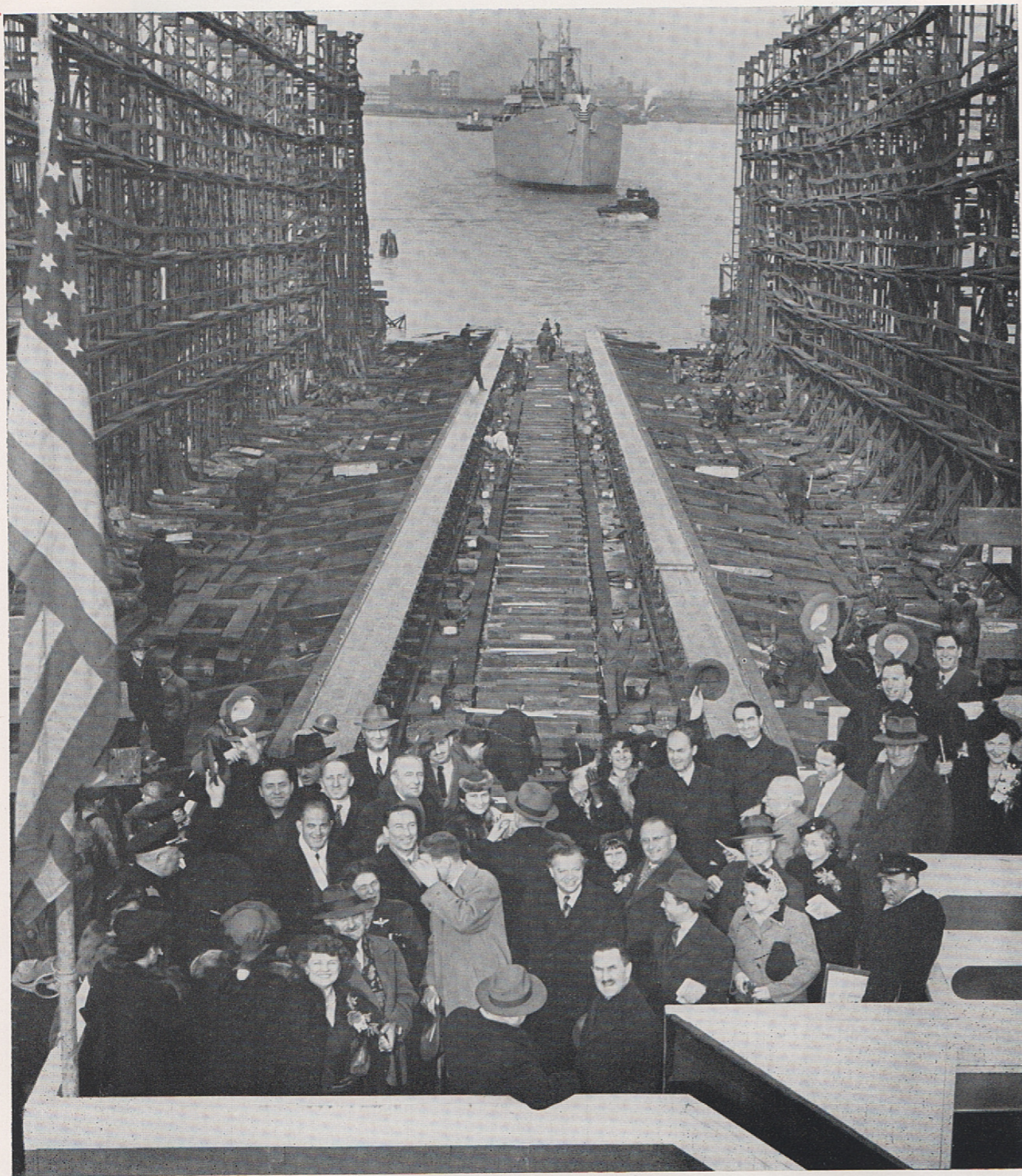
One of a half-dozen "Liberty Ships" built with funds realized from war bond purchases by ILGWU members and earmarked for that purpose during the war years—1942-45—glides down the runways at Baltimore into Chesapeake Bay. "D.D." is in the lower center with several associates, among them vice presidents Nagler, Feinberg, Zimmerman, Rubin and Kreindler, and Nathaniel M. Minkoff, secretary-treasurer of the Joint Board Dress and Waistmakers' Union.
