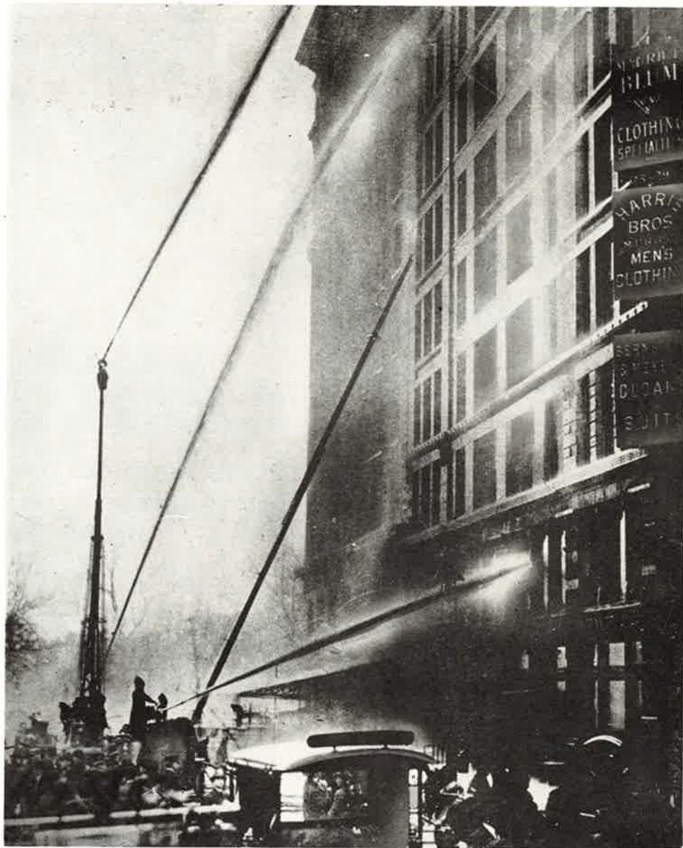
The water towers were of no avail. They reached only to the seventh floor.
